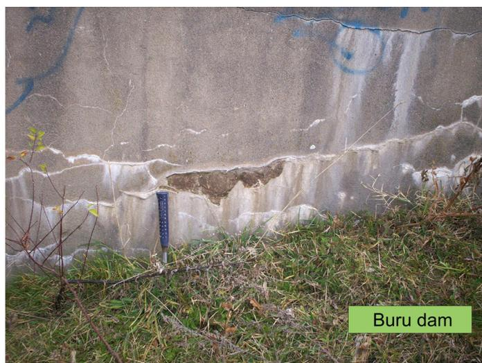
**Figure 1.** Fissures with carbonate deposits at the base of Buru dam (Cluj County).
